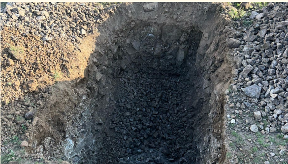
Recharge pits dug in low-lying areas of the field
