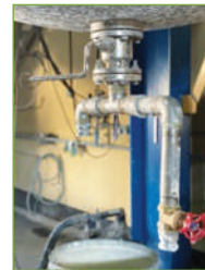
After installing T-Valve
